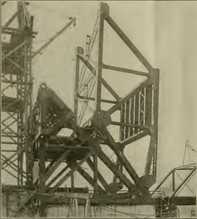
C & N. W. RY. DEERING BRIDGE—FIRST STAGE OF ERECTION. THE COUNTERWEIGHT PIVOT AND BASCULE SPAN PLACED READY FOR PERMANENT SETTING.
